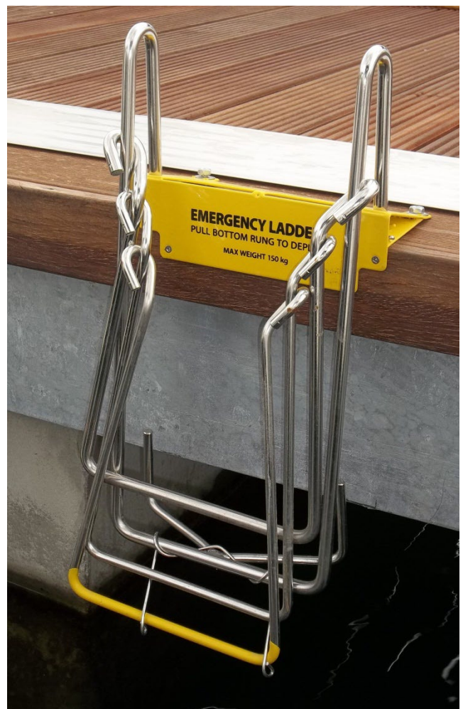
Figure 2. (above) The emergency ladders. Stored clear of the sea, they are activated by pulling on the bottom rung.
